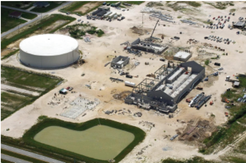
Figure 2: Construction Status for North RO Water Treatment Plant, Cape Coral, in September 2008
